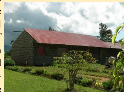
The new building is almost finished!
